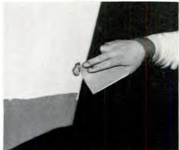
GOUGE is then sanded with 100-grit sandpaper to remove dirt and provide roughened surface for putty
